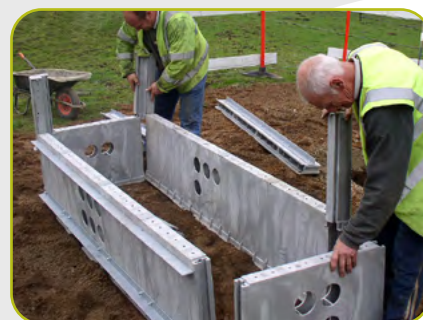
Assembly of a RADBOX chamber
