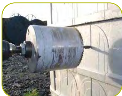
Creation of cable pipe entries
