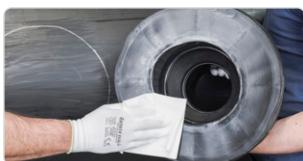
**6. Unpack the product from the bag, degrease the pipe and lower welding part of the fitting with the PE pipe cleaner recommended by the manufacturer, allow the liquid to evaporate completely, do not touch the prepared surface**
