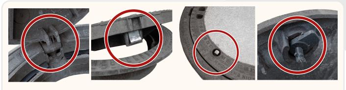
Inspect all moving components, for instance, hinges, screws and screw fastenings, locks, and springs.
