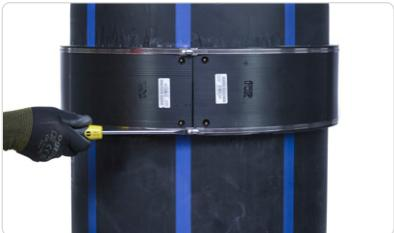
**5. Put two parts of repairing patch on the pipe and hold them with two metal clamps**
