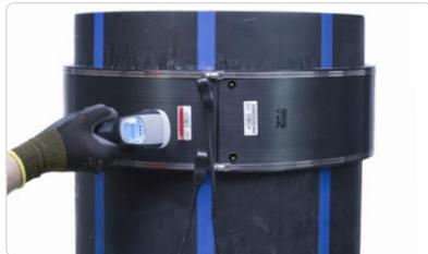
**6. Start welding and proceed according to the requirements of the machine**
