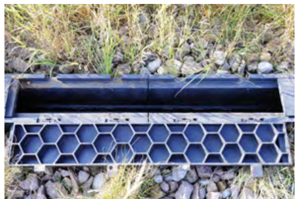
Convenient access to the cables!
