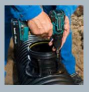
4. Push in the connecting socket and fix it with bolts.
