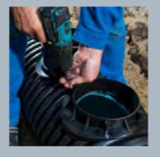
2. Fasten the groundplate on top of the pipe.
