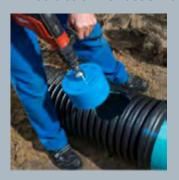
1. Drill a hole into the pipe.
